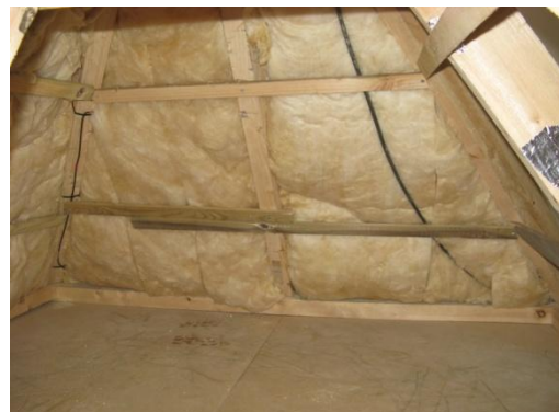
Fig. 2 An image from inside showing glasswool applied on rafters
