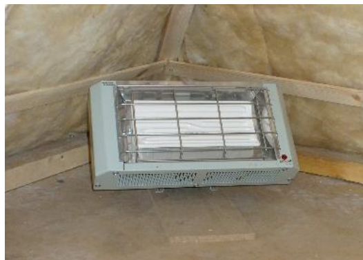
Fig. 8 Ceramic heater in position
