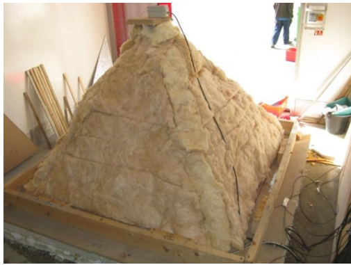
Fig. 3 Glasswool applied over rafters
